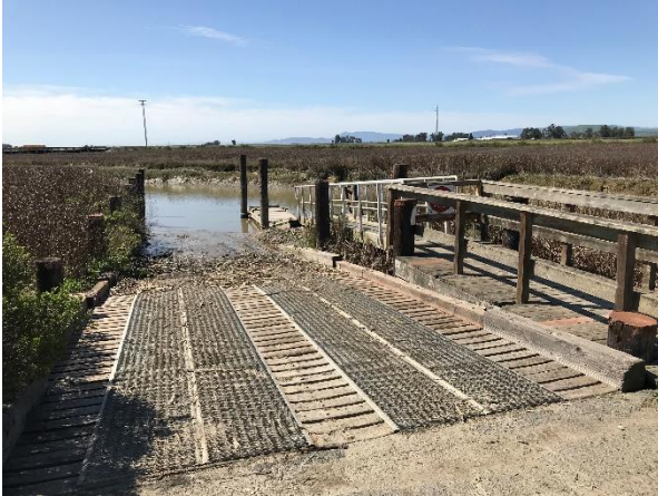
Boat Ramp & Pile-Guided Boarding Float
